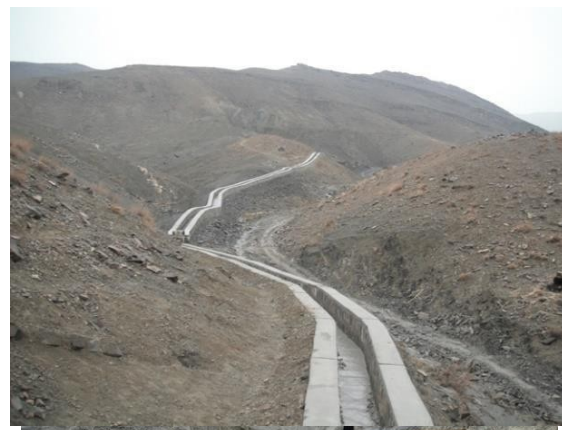
Figure 3: Newly constructed water channel
